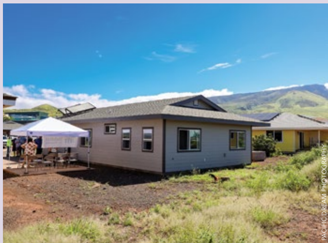
Habitat for Humanity Maui's first home rebuild
